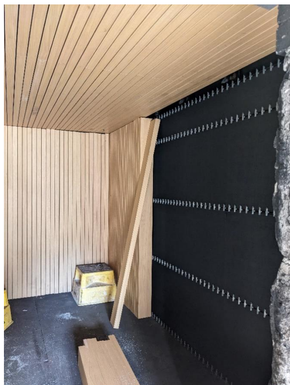
Figure 1 Partial Installation of Test Specimen FI18182-02-1
